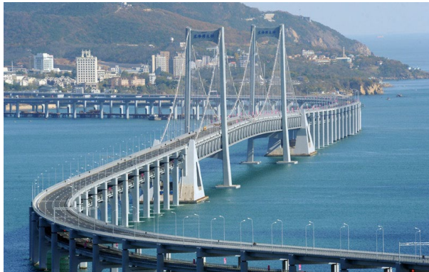
Xinghai Sea-across bridge
