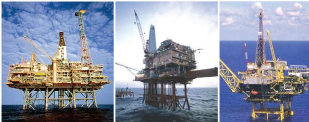
Fig. 1. Oil platforms basing on spatial beam supporting structures
